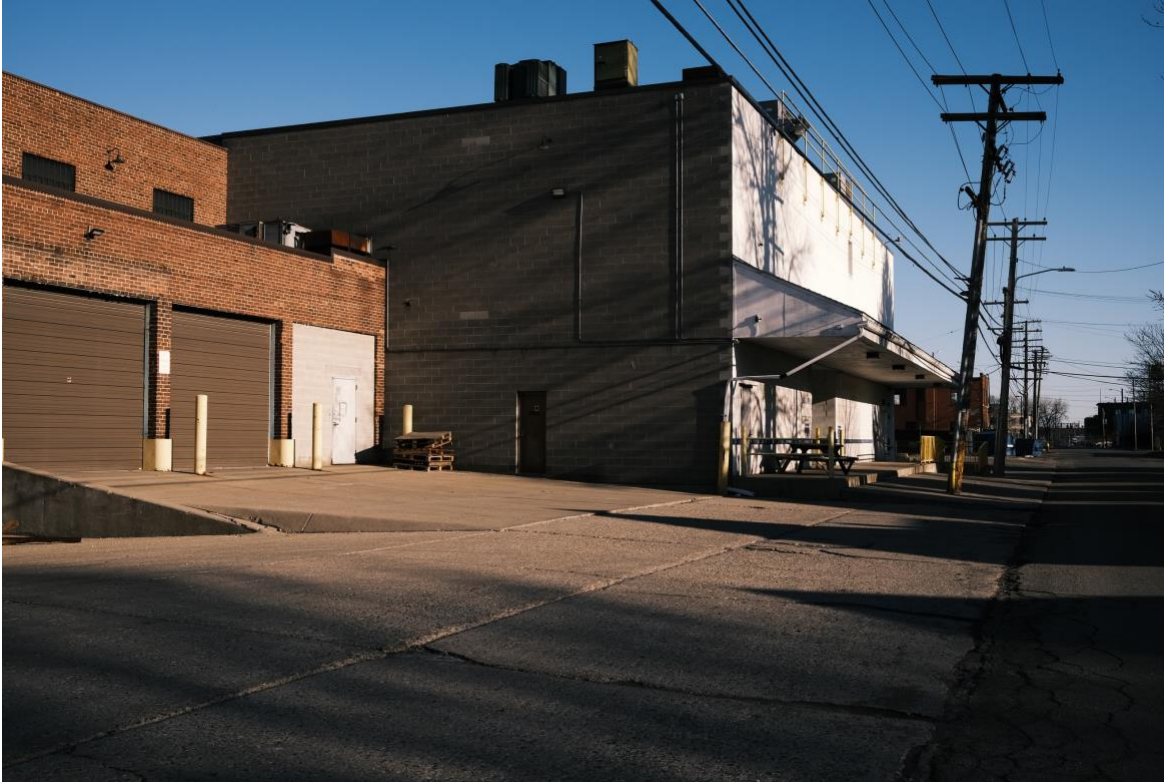
Figure 23 Industrial buildings directly across from single-family homes [next photo]
