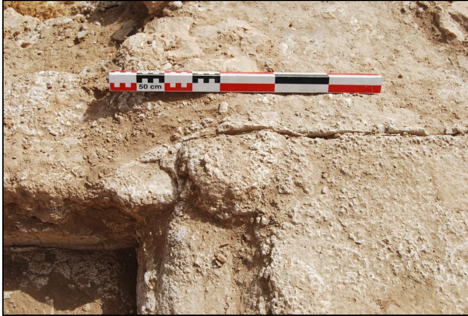
Figure 95: Northeast corner of installation showing it was a separate construction from the wall and the door jamb to the immediate left.
