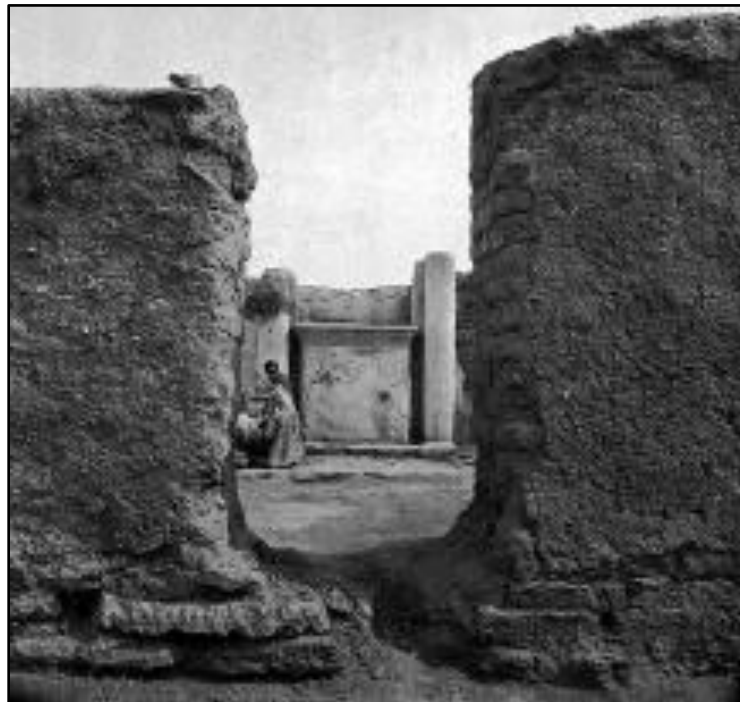
Figure 41: Room 7W in the Temple to Azzanathkona looking east as photographed between 1931 and 1933
