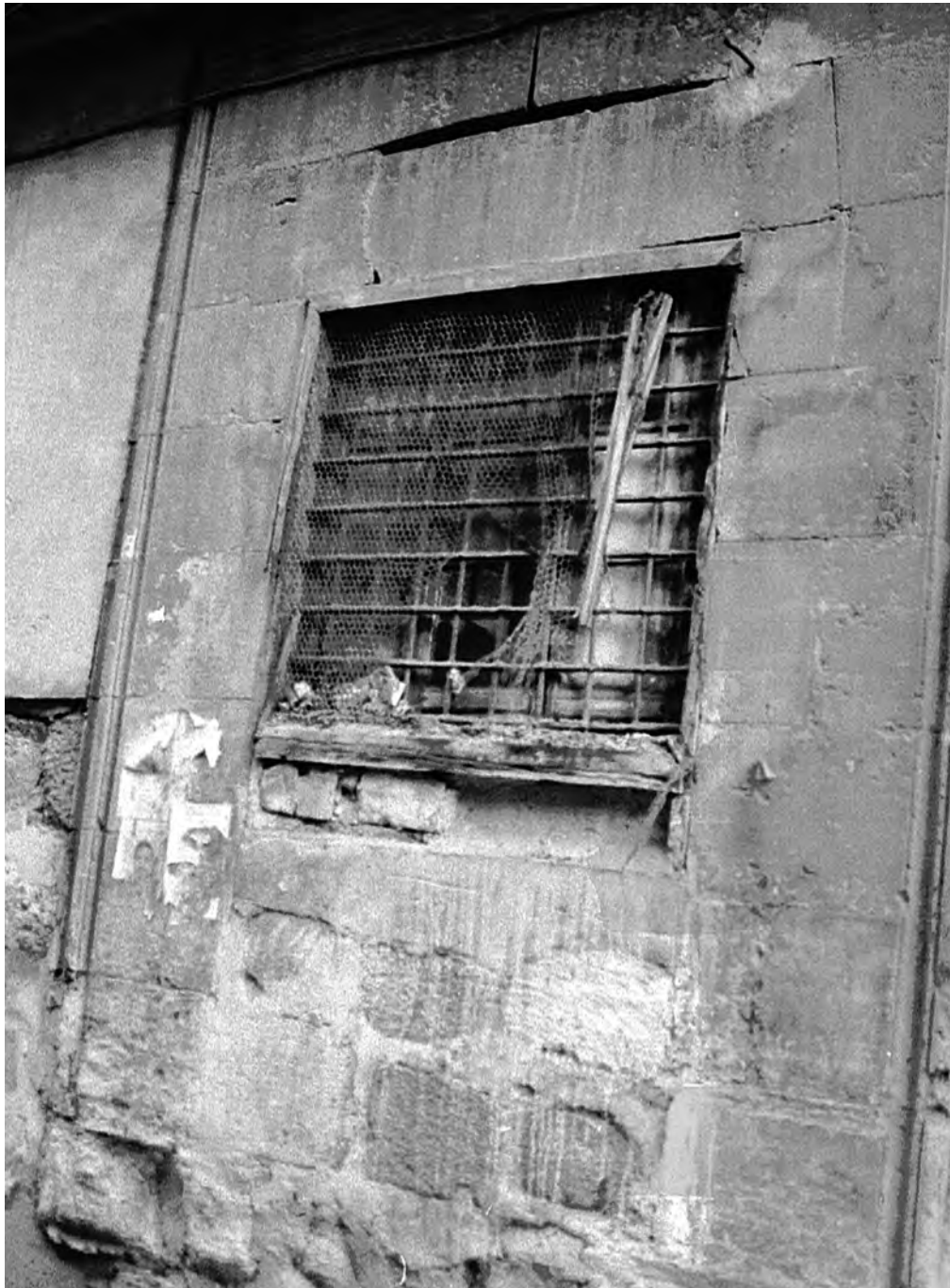
Fig. 8. Damascus, Tankizīyah: east façade, large window
