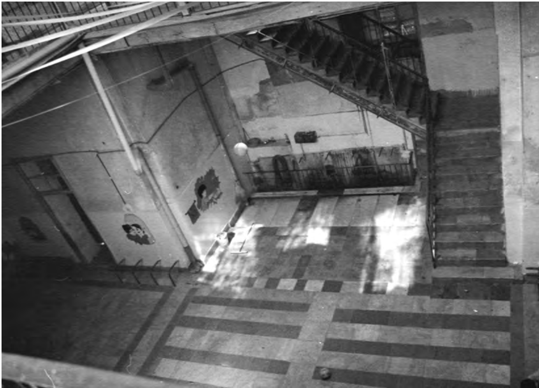
Fig. 11. Damascus, Tankizīyah: interior, view of east īwān
