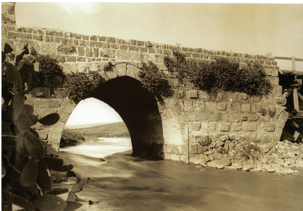
Figure 11b. Bridge, from southwest, with second arch under repair, 1919. Note Crusader masonry between arches. L. A. Mayer Collection, The Hebrew University of Jerusalem, Dept. of Islamic and Middle Eastern Studies (Mayer_30A).
