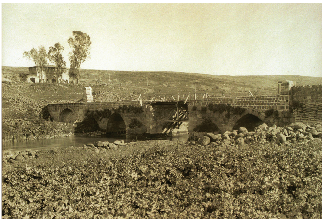
Figure 3. Banāt Ya'qūb Bridge under repair, 1919, looking southeast. L. A. Mayer Collection, The Hebrew University of Jerusalem, Dept. of Islamic and Middle Eastern Studies (Mayer_28A).
