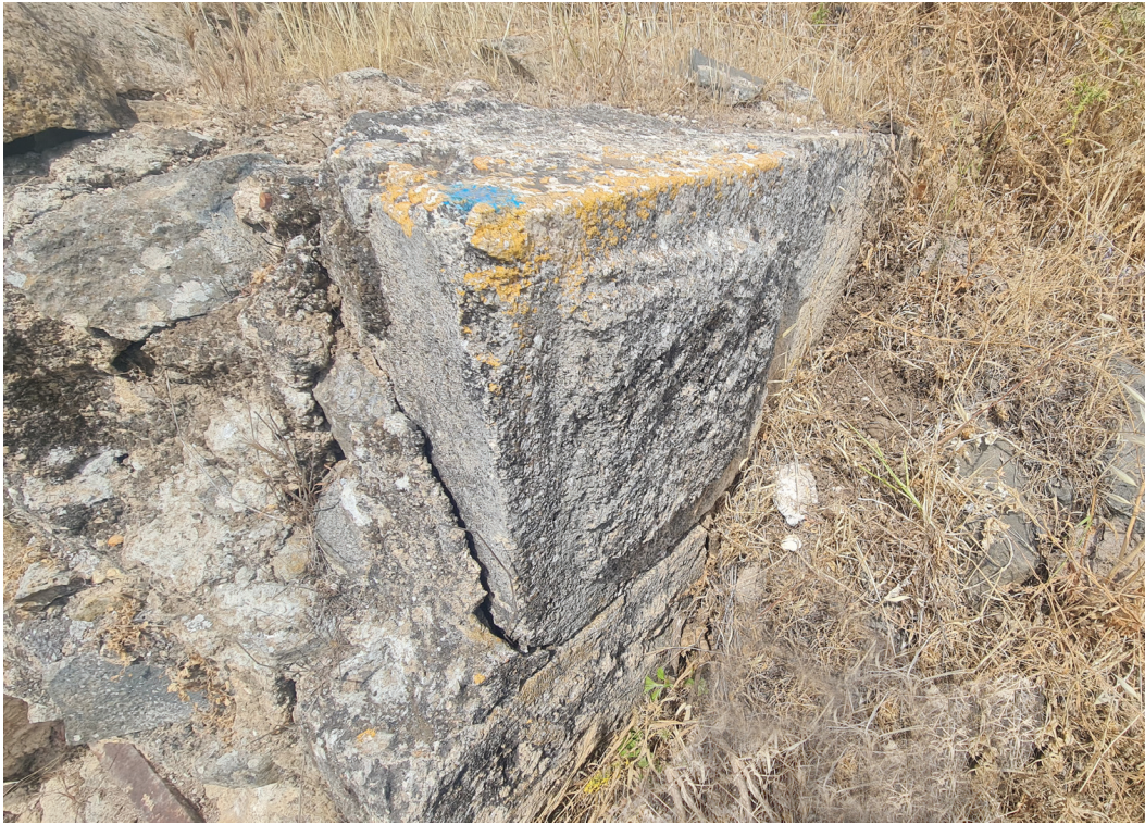
Figure 12. Detail of drafted masonry, likely of Crusader origin, on the surviving section of the east bank bridge, looking north. Photograph by Katia Cytryn, May 21st, 2021.
