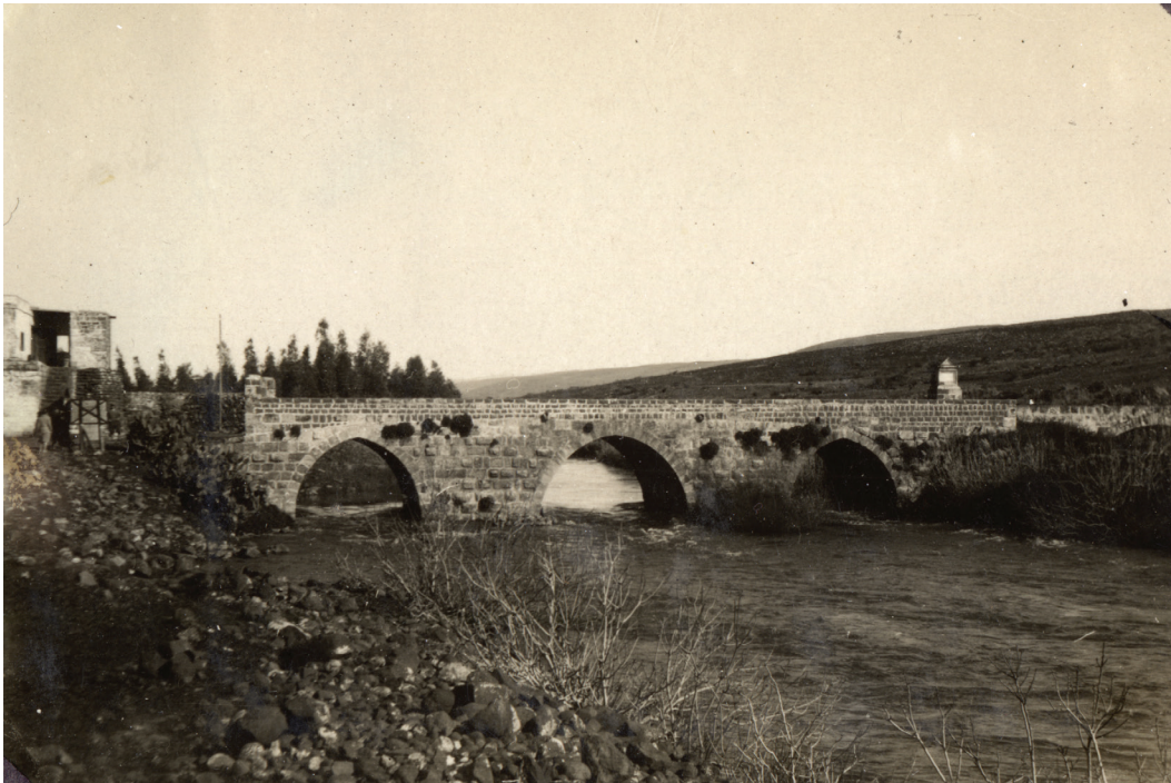
Figure 10. Bridge, with second arch from west (originally middle arch) repaired, January 1929. From Bohman Max Collection, Shoshana and Asher Hal- evi photo archive. Yitzhak Ben Zvi (YBZ_0358_336).
