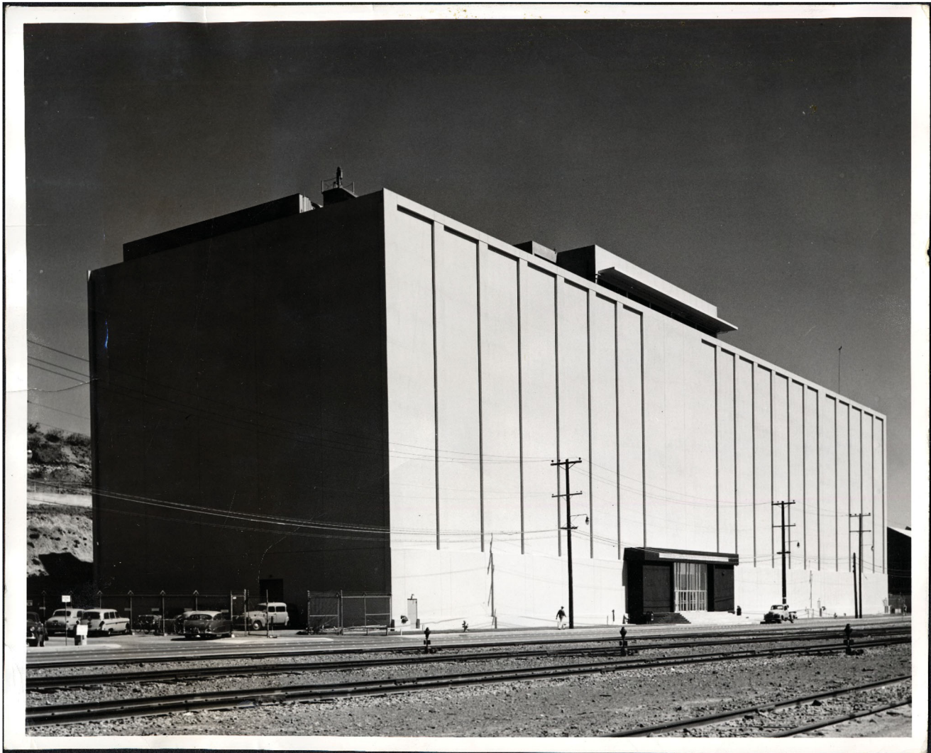
Figure 5. US Naval Radiological Defense Laboratory building at HPNS (Unknown 1955).
