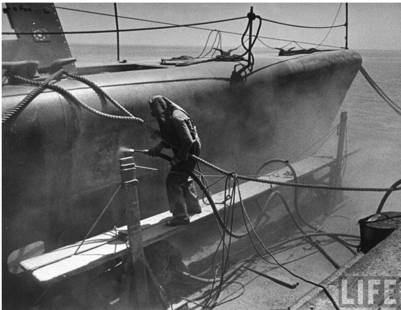
Figure 4. Sandblasting of Naval vessel at HPNS to remove radionuclide contamination (circa 1947) (Art House SF 2019).
