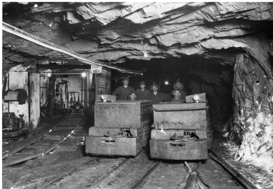
Figure 5. Electric Storage Battery Locomotives in a Republic Mine drift, 1920. 70
