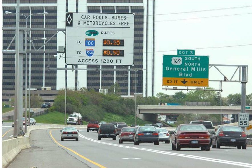
Figure 1.1: Snapshot of highway I-394, Eastbound direction, just before the exit to General Mills Boulevard. The Express Lane is the leftmost lane, separated by the rest of the highway by a double white line on the ground. Source: Buckeye [2012].
